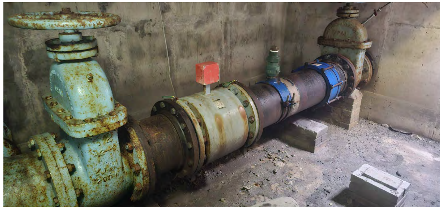
EXISTING METER VAULT INTERIOR
