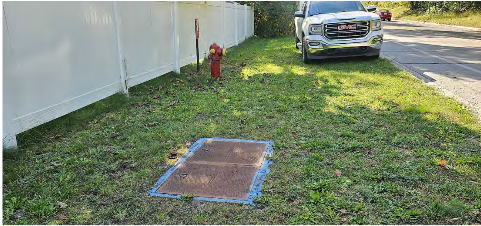
EXISTING METER VAULT HATCH
