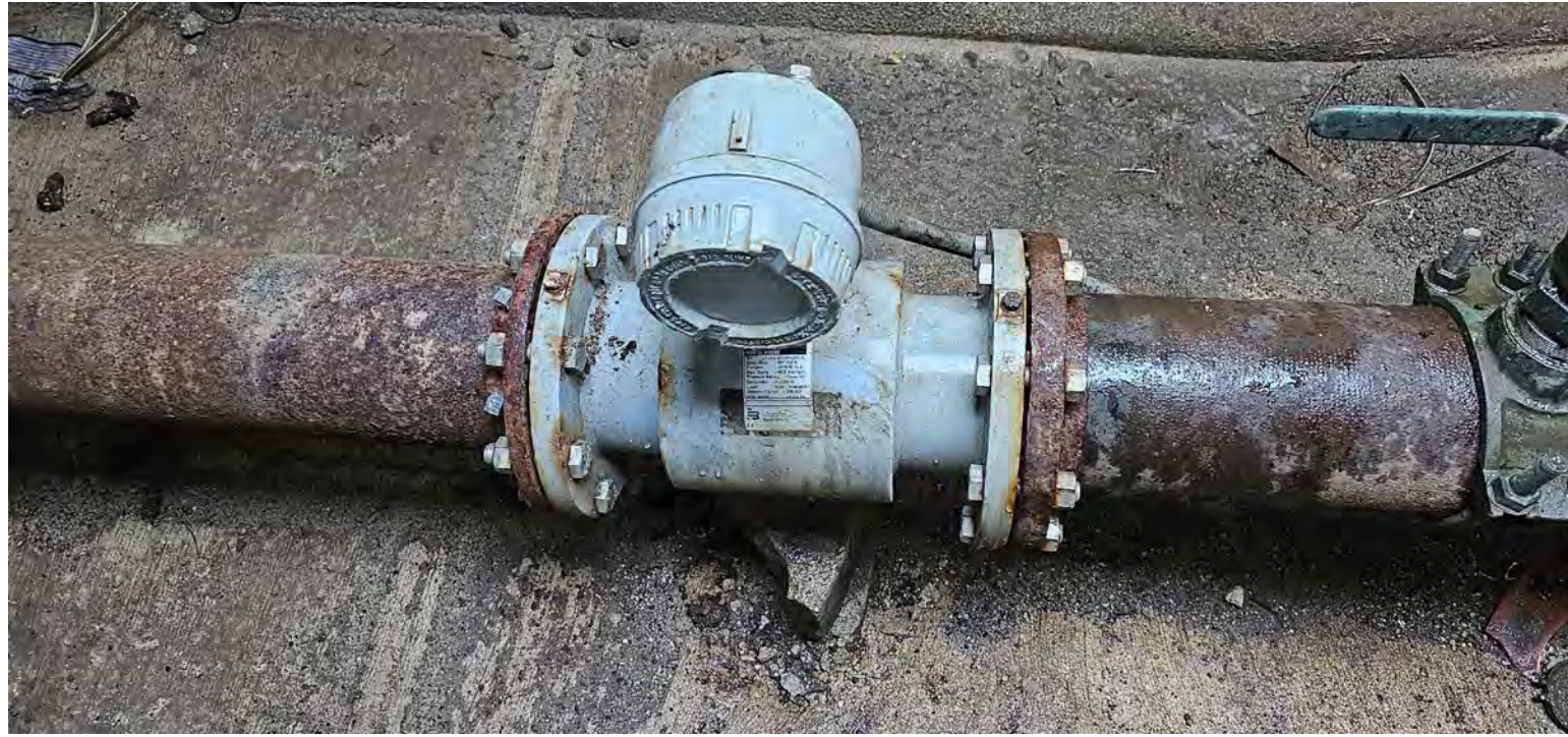
EXISTING METER VAULT INTERIOR
