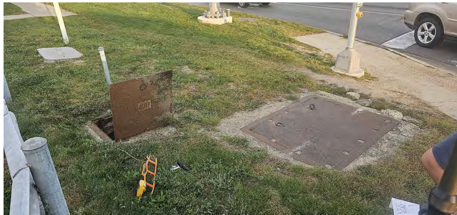
EXISTING METER VAULT HATCH
