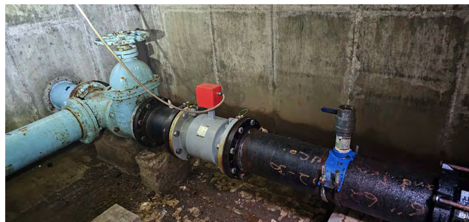
EXISTING METER VAULT INTERIOR
